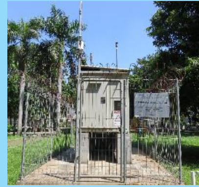
DK1 in a residential area in North Jakarta
